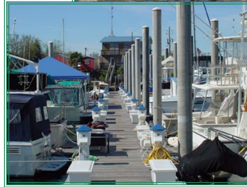
The photo on the top shows Mahogany Marina after it had been devastated by Hurricane Ivan in 2004. The docks and 43 of the 50 boats at the marina were completely destroyed. The rebuilt facility, renamed Palm Harbor, shown in the bottom photo, was tested the following year when the eye of Hurricane Dennis, a Category 3 storm, passed within 20 miles. There was no damage to the docks or boats.
