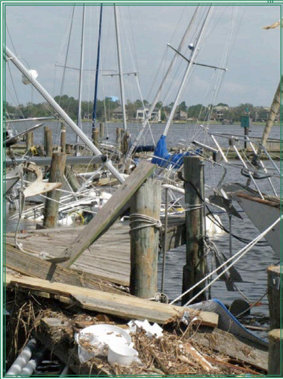
The single most important determinant in how well a facility will fare in a storm is its location. A marina that is only protected from open water by a two-foot-high seawall, like the one shown on the left, will need a far different plan than one that is surrounded by land, like the one on the right. The photos of the two marinas—Watergate Yachting Center and the Waterford Harbor Marina—were taken several days after Hurricane Ike had passed over the area.
