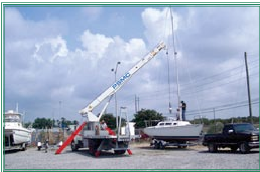
PSMC, Jacksonville, Florida: Using their portable crane, masts can be pulled fairly quickly—in as little as a half hour if the electrical wiring harnesses are disconnected and turnbuckles loosened.
