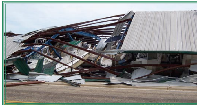
Older buildings have proven to be especially vulnerable. This one went over in Ivan.
